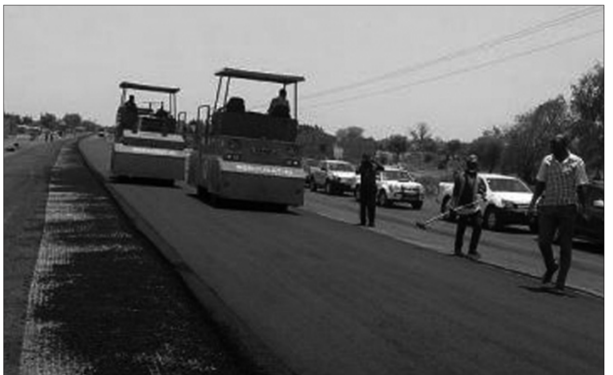
Road construction funded by AFD
