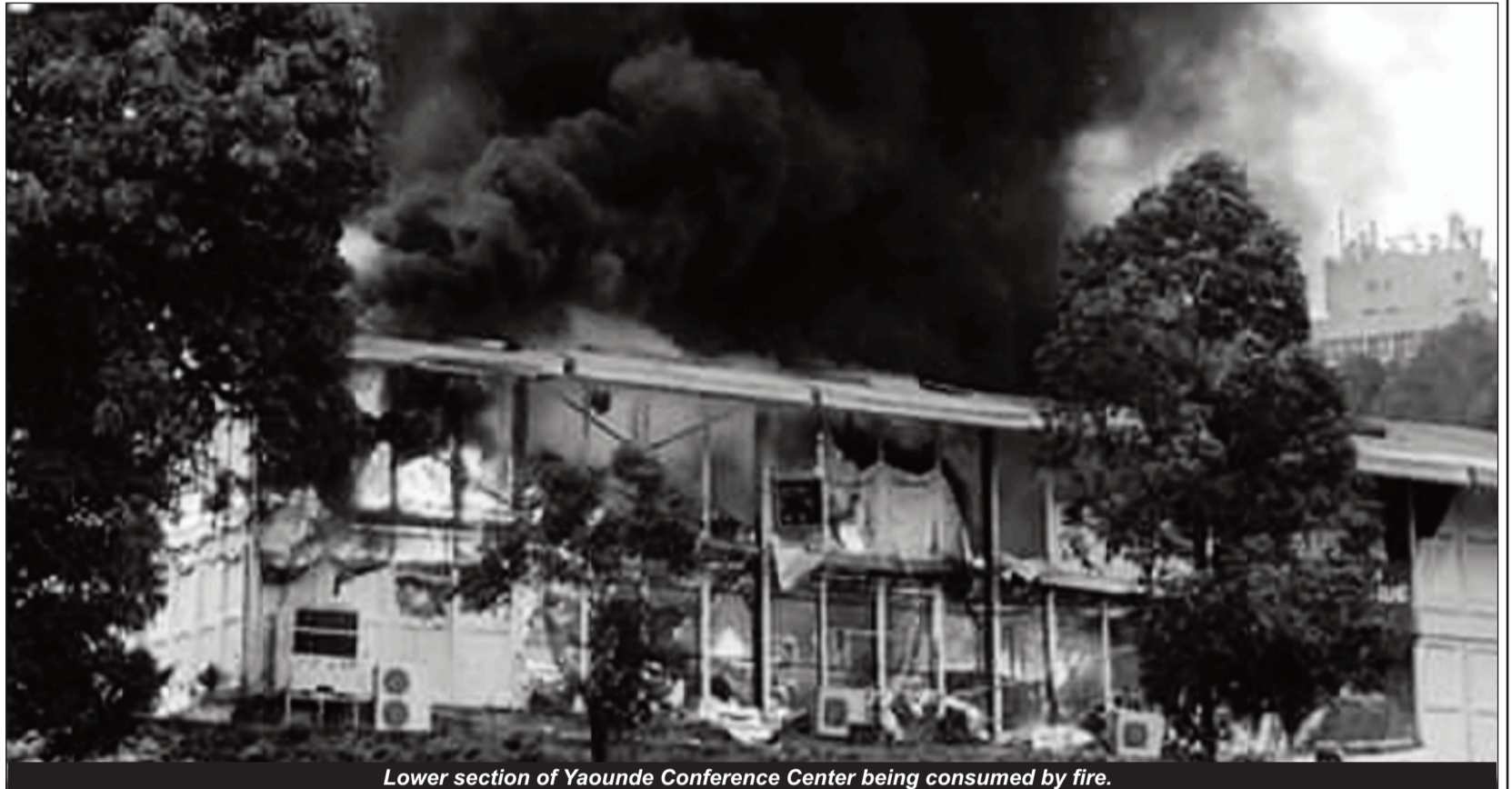
Lower section of Yaounde Conference Center being consumed by fire.
